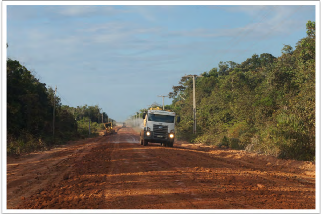
Figure 6 – Maintenance work being executed in May 2018. Photo: author
